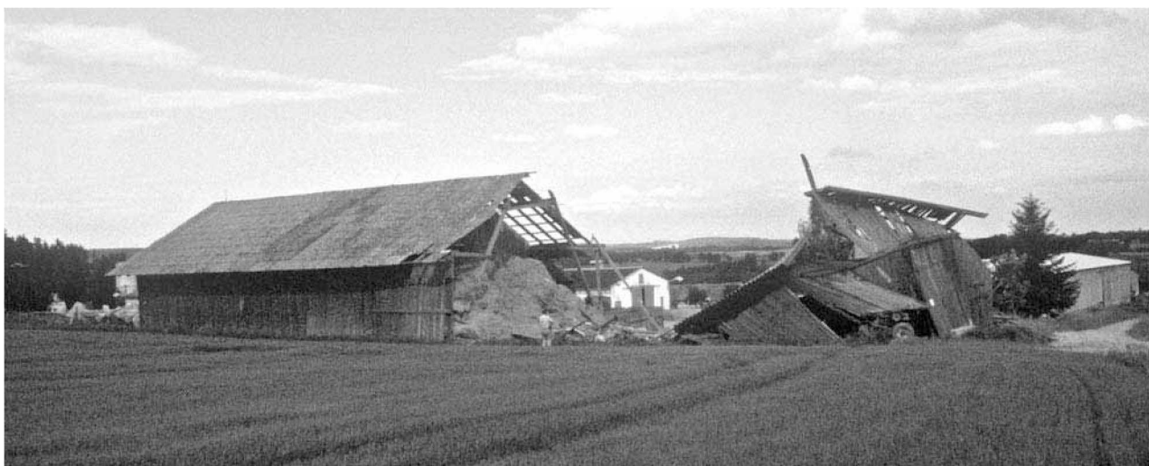
Fig. 7. A barn (close to Mrzkovice village) partially damaged by a smaller tornado. The tornado passed through the right side of the barn, while the left part remained intact. Photo by M. Setvák.
